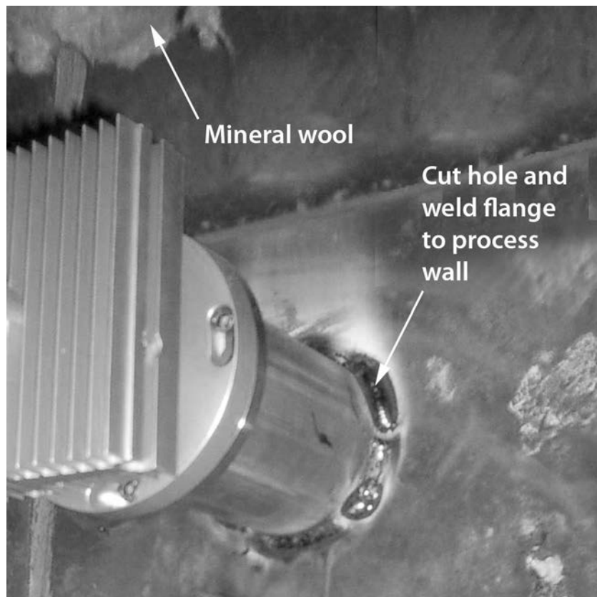
Figure 82 Cooling Set Installation
